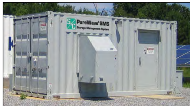
Figure 6-2 – Typical 1.25MVA containerized PCS from S&C electric company
