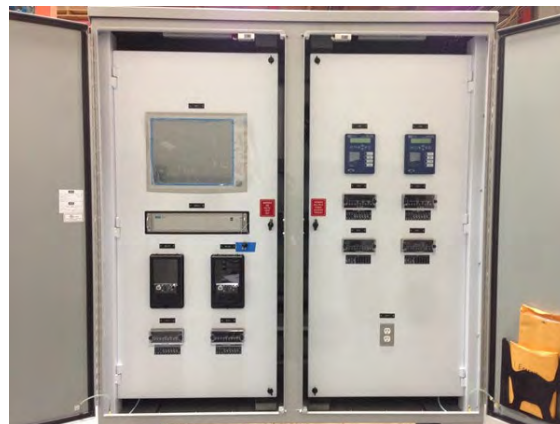
Figure 6-5 – Typical control cabinet
